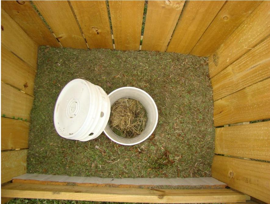
Pour your cut vegetation around the bucket and raise the bucket as you fill the compost tower over time. A four foot wide by three foot deep by four foot high tower will take about a half a year to fill if the toilet is being used daily by two people. It is important that the level of the waste and the level of the composting vegetation remain the same. Allowing the surrounding vegetation to rise higher than the waste inside will generate too much heat and will be lethal to the BSF larva.
